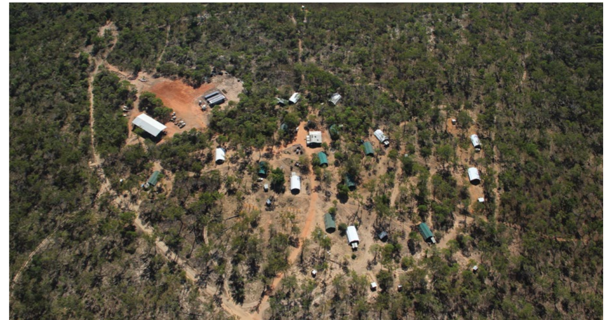
TOP: Aerial shot of Kabulwarnamyo, headquarters of Warddeken Land Management Ltd. Kabulwarnamyo is a unique community built and maintained by rangers, largely without government funding. BOTTOM LEFT: Eikanah Dullman, Matthew McClaren and Chris Bald work on construction of the first house at Kabulwarnamyo. The house is being built using funds generated by Warddeken through the sale of carbon credits. BOTTOM RIGHT: Rangers camp out and undertake maintenance at the remote Makkalarl balabbala safari tent. Photo by Rowand Taylor
